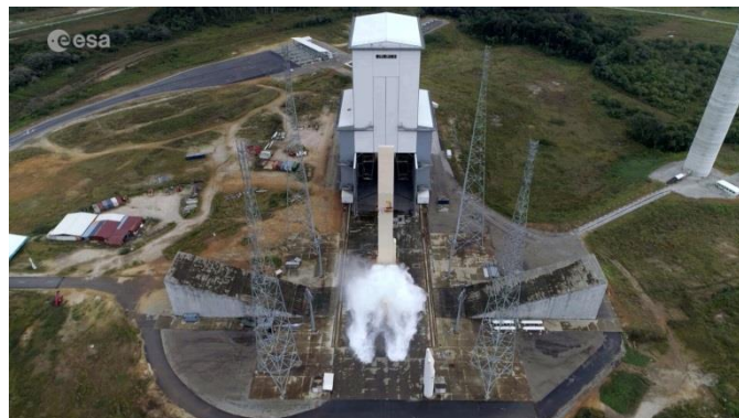
Ariane 6 launch pad water deluge system test
