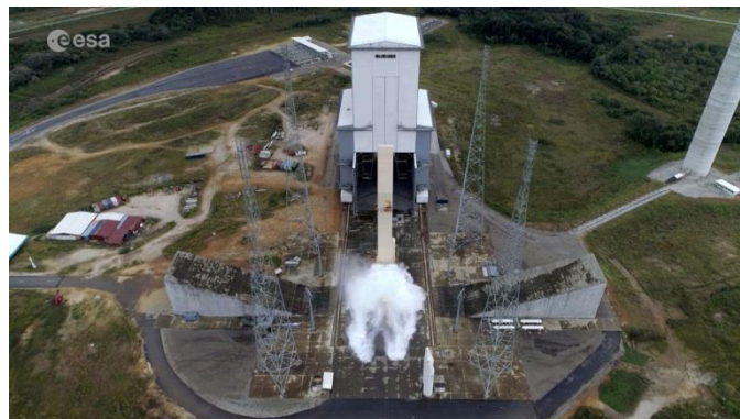
Ariane 6 launch pad water deluge system test
